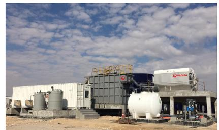
**Veolia Water Technologies Qatar** was contracted by Baladna, Qatar's leading dairy producer, to upgrade the existing wastewater treatment facility at its cow farm located in Al Khor, north of Doha. Veolia proprietary technologies will allow an increase in the treatment capacity of the plant and enable the treated wastewater to be reused for agricultural irrigation purposes.
